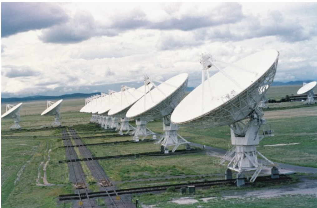
Figure 4: Typical radio astronomy site located in Socorro, NM (Image courtesy of NRAO/AUI)
